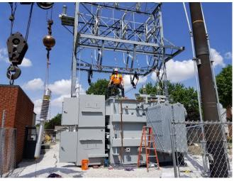
CRMU's contractors are nearing completion of our major substation capital improvements. In the picture to the left you see contractors completing the transformer assembly—as they are finishing the installation of the high side bushings and radiator fins on the transformer
